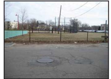
No sidewalk on Holly Street (3F)
