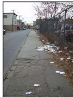
Spruce Street Sidewalk (1H)
