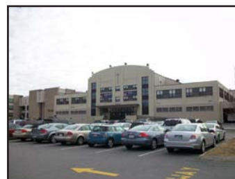
Central Catholic High School Parking Lot (3A)
