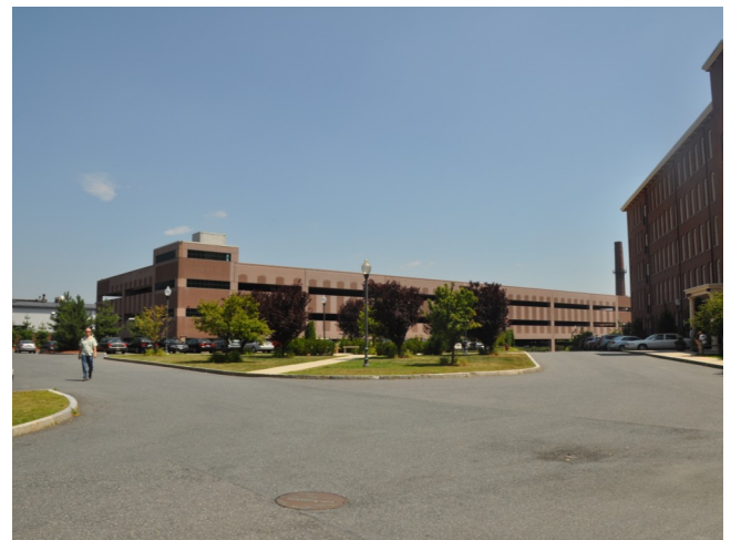
The 5 story shared parking lot for the adjacent developments.
