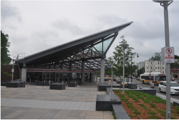
Renovated Ashmont MBTA Station, 2011.
