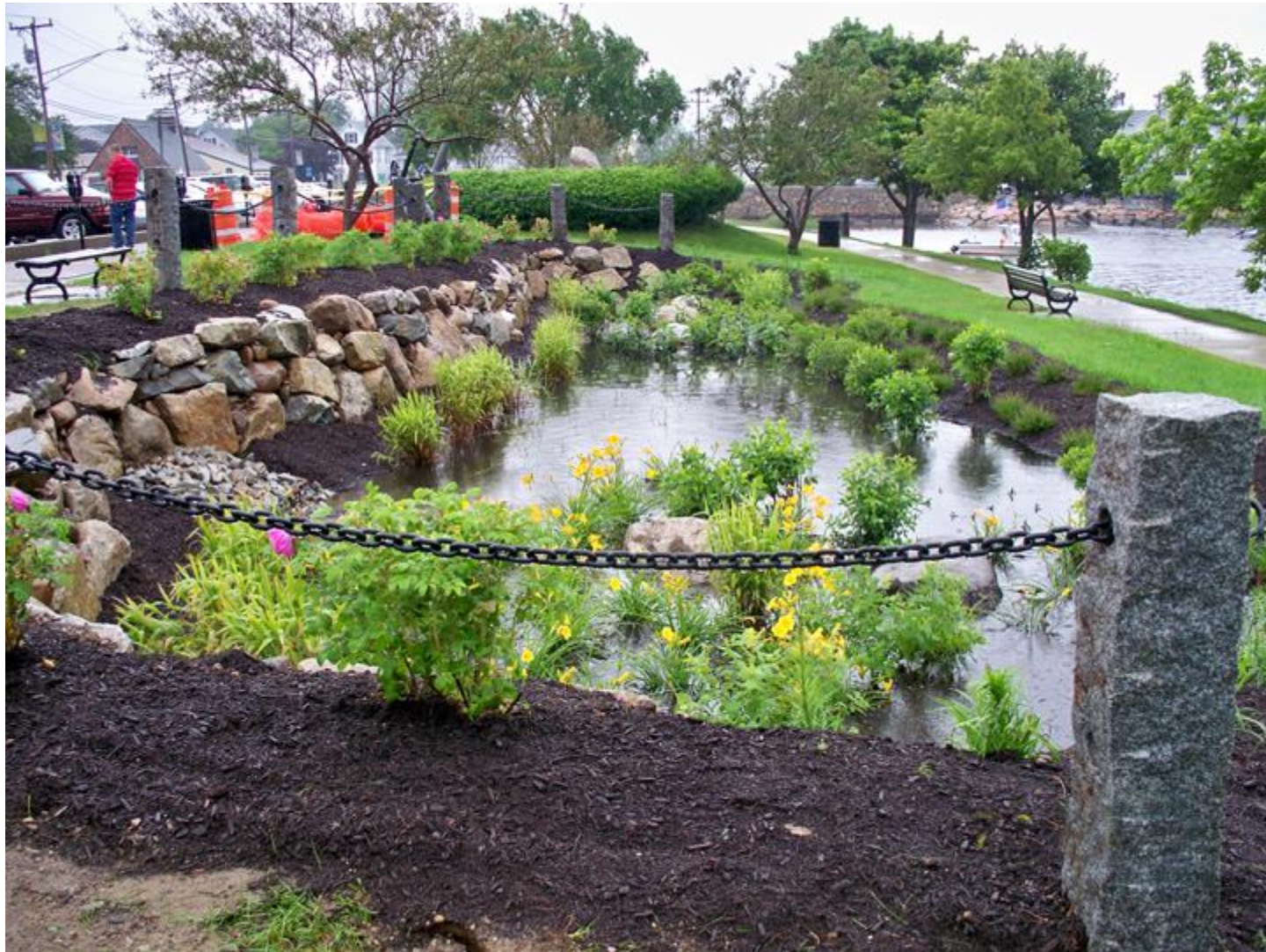
Bioretention Cell Water Street, Plymouth Center, MA
