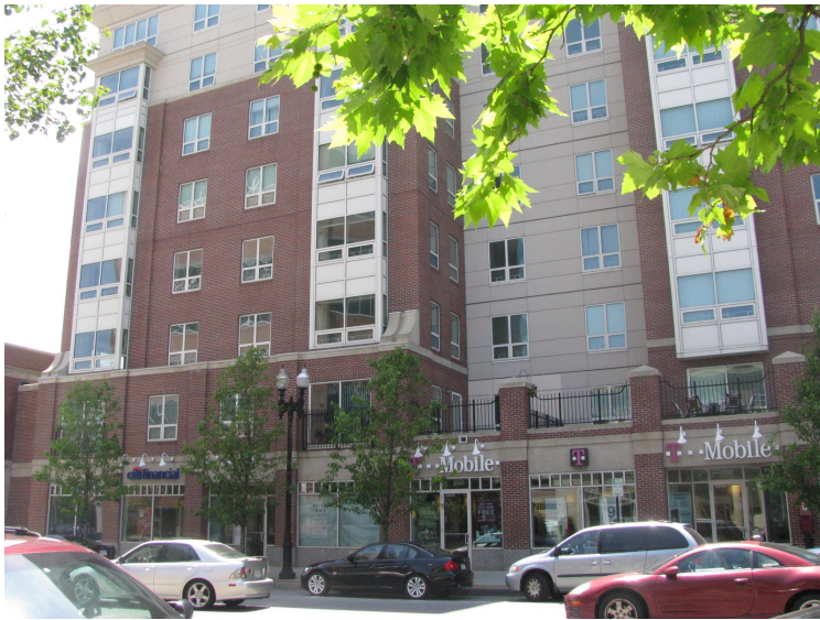
View of Mixed Use on Hancock Street at Quincy Munroe Place
