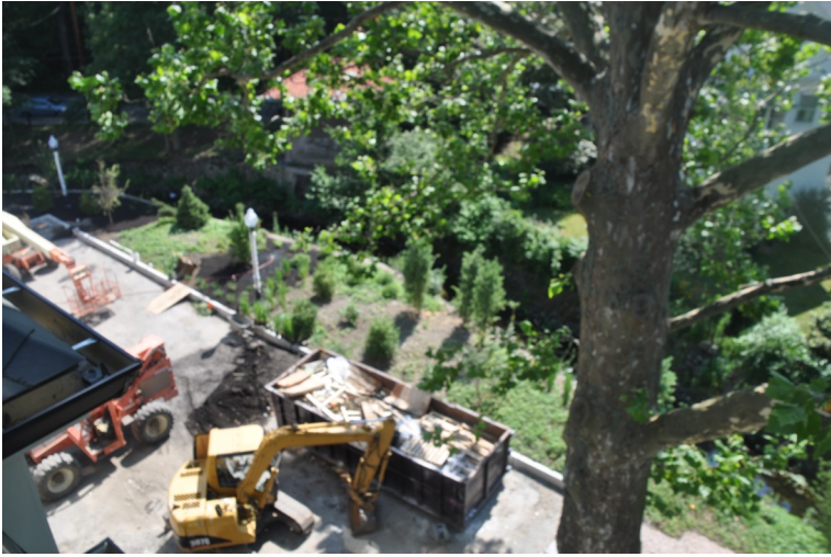
Construction of parking spaces and community space in the back of the development, 2011.
