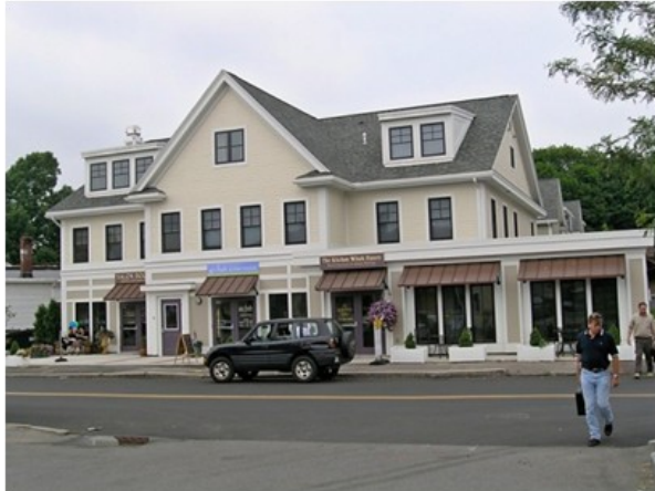
Summer Street Retail with apartments above. Source: Affirmative Investments, 2009.
