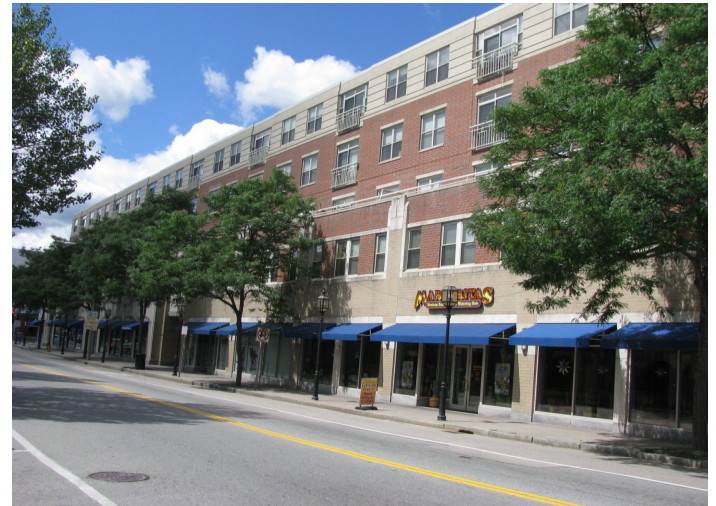
Apartments with ground floor retail and restaurants. Cronin's Landing, Moody Street, Waltham, Ma.
